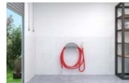
Wall fixings in garages
